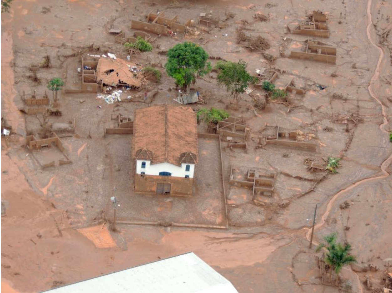
Figure 5 Church after the collapse of the Fundao dam, Brasil (Source: patrimoniocultural.blog.br ).
